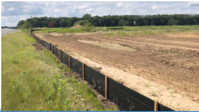
PROPER SILT FENCE INSTALLATION
