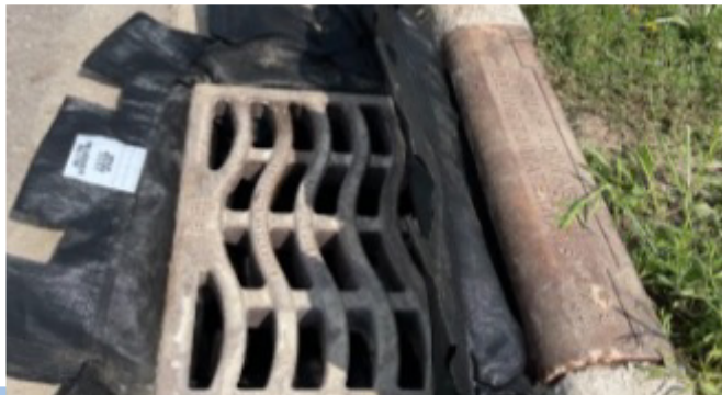
PROPER CATCH BASIN INLET PROTECTION
